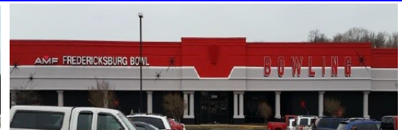
AMF Fredericksburg Lanes
